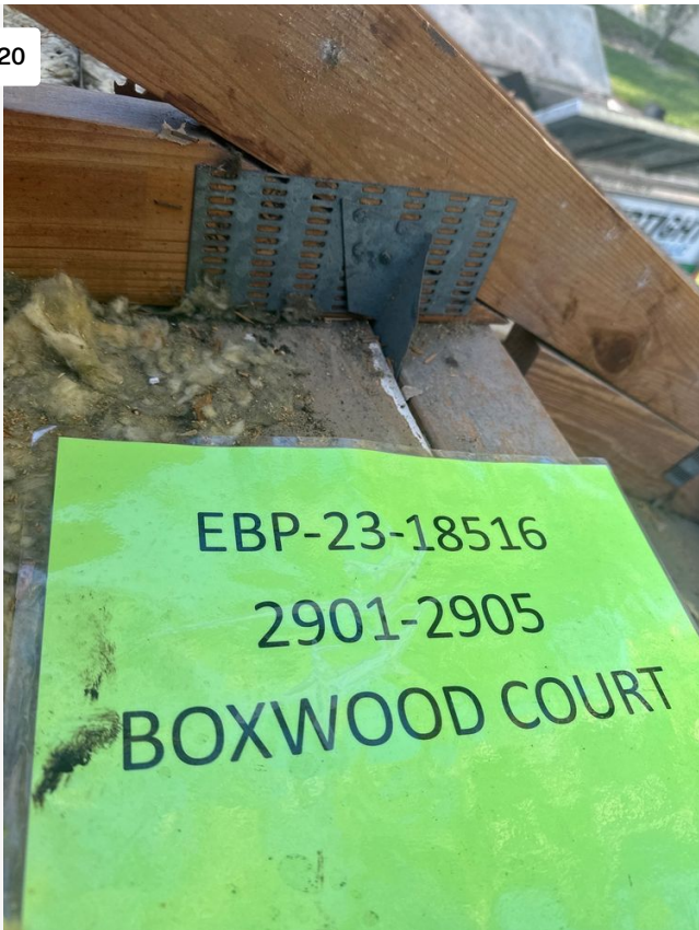
Project: 2901 Boxwood Ct Date: 11/20/2023, 4:03pm Creator: Maynor Perez
